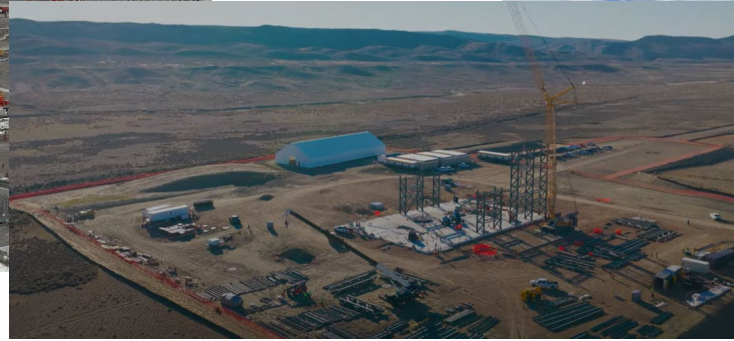
Terrapower Natrium – site preparations, sodium facility construction underway in Wyoming
