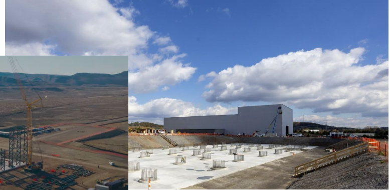
Kairos Hermes – drilled piers installed in Tennessee
