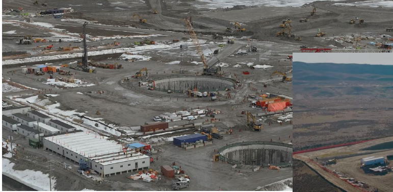
OPG/Darlington GE-H BWR X-300 early site works completed in Ontario
